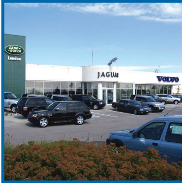
Front glass before Sunscape was installed
