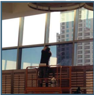
In progress; Starlite 18 on lower half of windows
